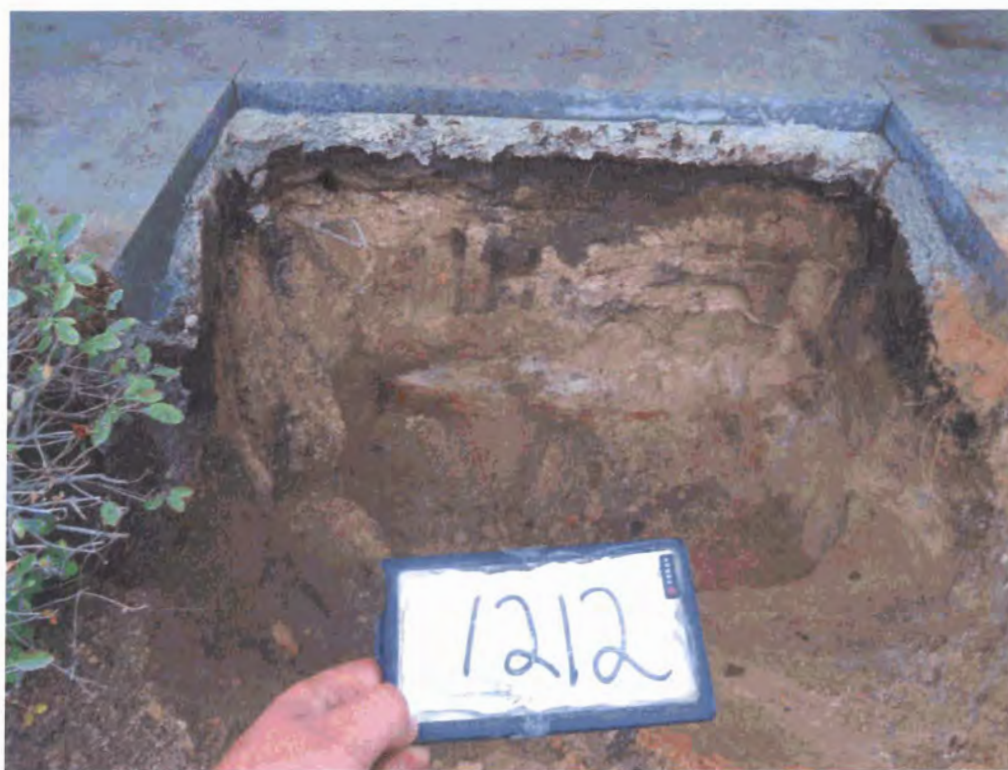
Picture 2: UST 1212Cardinal excavation.
